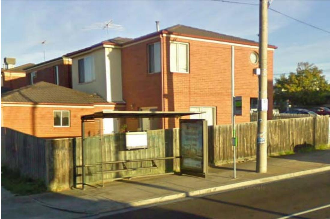
**Image 2:** This advertising shelter has been installed incorrectly blocking both sides of entry to the shelter by a person using a mobility aid or a person with vision impairment. The Tactile Ground Surface Indicators have also been installed incorrectly. Standards 18.3 state they need to be a contrasting colour.
